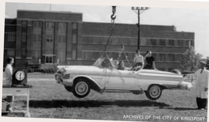
The original caption for this demonstration of the product then known as Eastman 910 Adhesive said it supported a weight of more than 2 ½ tons based on a 3.15-square-inch, steel-to-steel bond.
